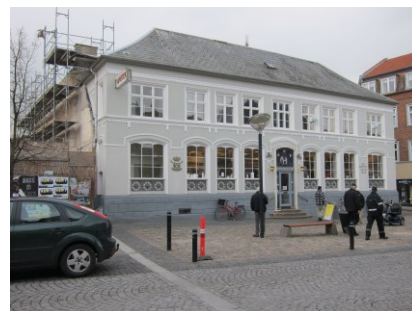
Facaden mod Ahlgade
